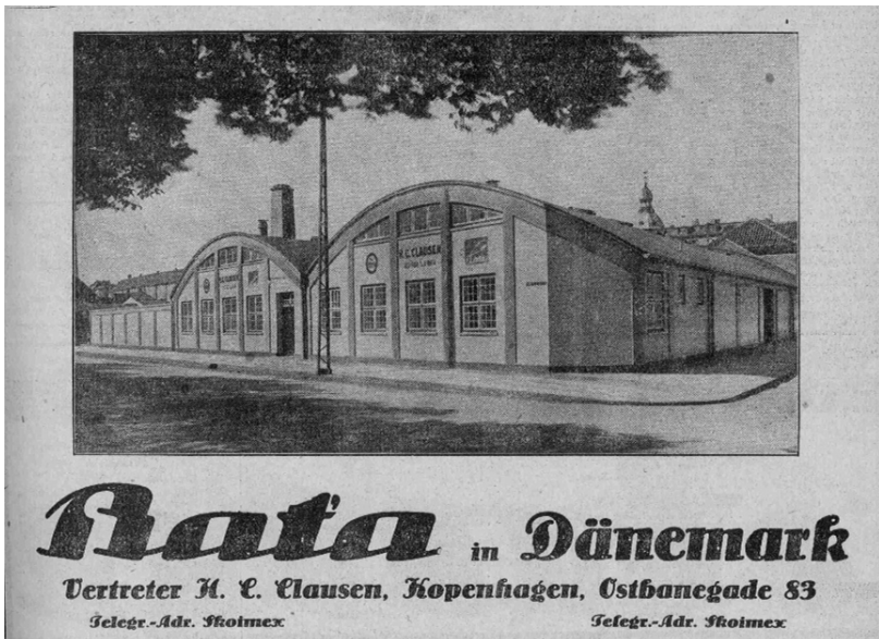
COMPANY REPRESENTATIVE IN DENMARK | 1926
